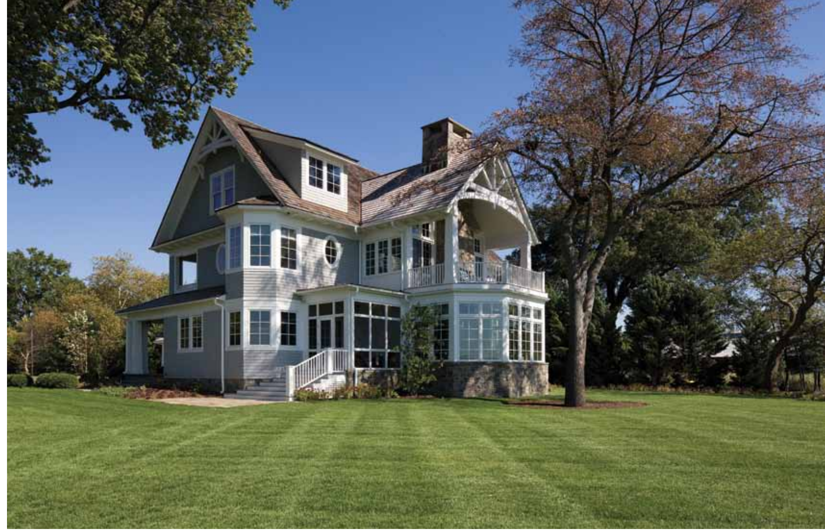
Top and Below Right: Painted white mahogany trim, wood-shingled roof, timber-truss details, stained wood shingles and a stone veneer base are custom features that add texture and warmth to this home.
