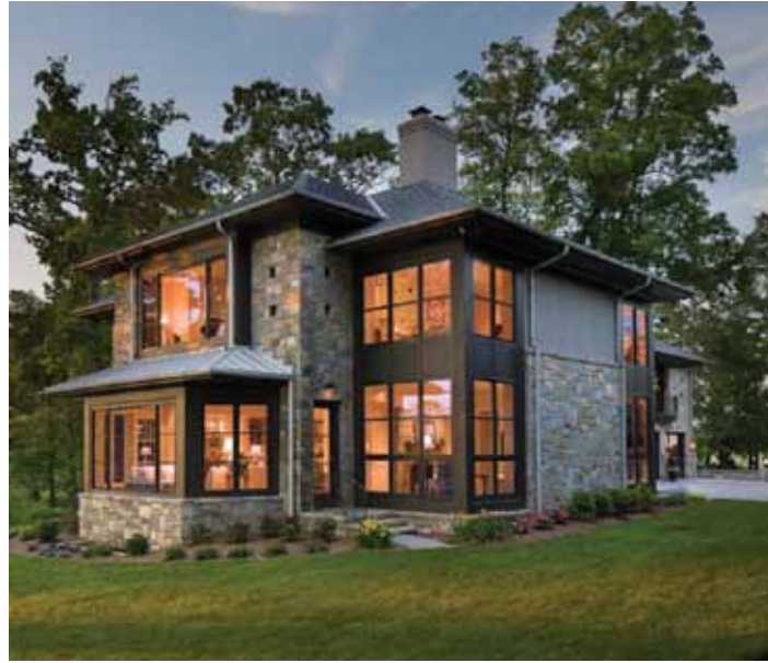
Above: A home on Mill Creek is clad in stucco and stone, with Marvin windows and galvanized gutters/downspouts; portal openings in the stone admit just the right amount of light into the home. Below: The crisp, white-painted open-plan kitchen/family room of a traditional home is enhanced by extensive millwork and coffered ceilings.
